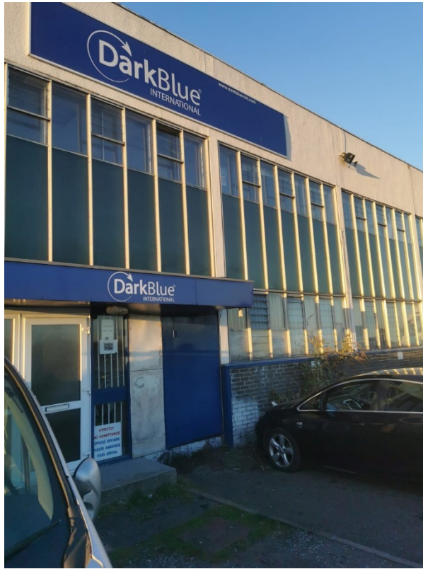
Image 3 - Current Frontage of LDN Riverside Unit
