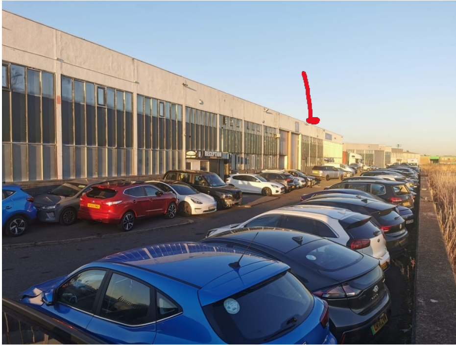
Image 4 - View of entire industrial building - LDN Riverside far end.
