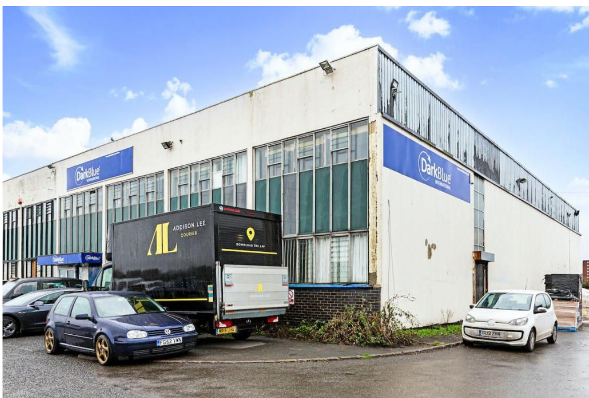
Figure 2: External view of building
